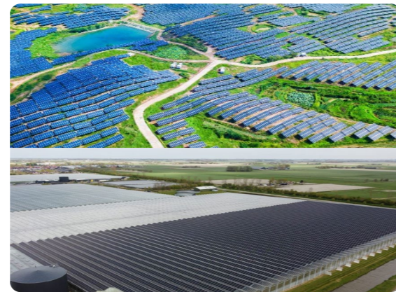
Agri-PV solutions applied in open fields and greenhouses
